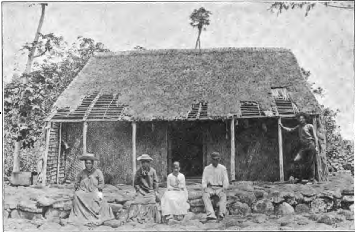
FIG. 84. HOUSE IN PUNA, WITH LANAI.
